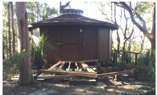
Repair work in progress
