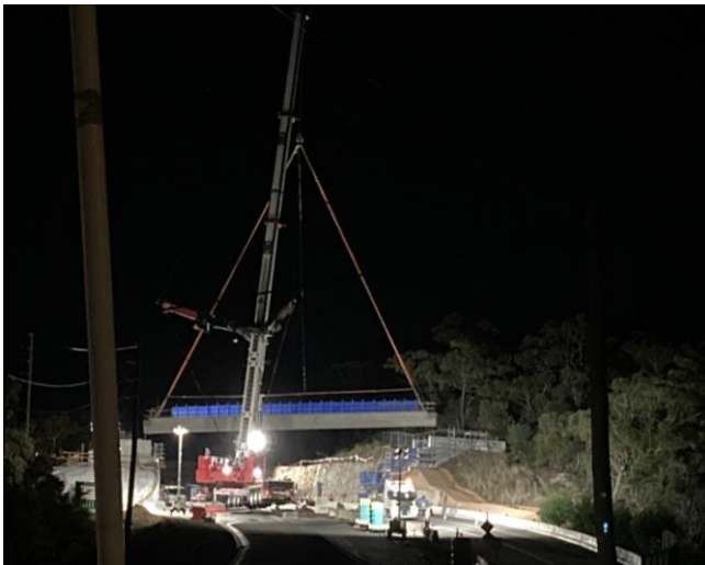
A crane was used to lift the bridge beam into position (Photo – Marita Macrae)
