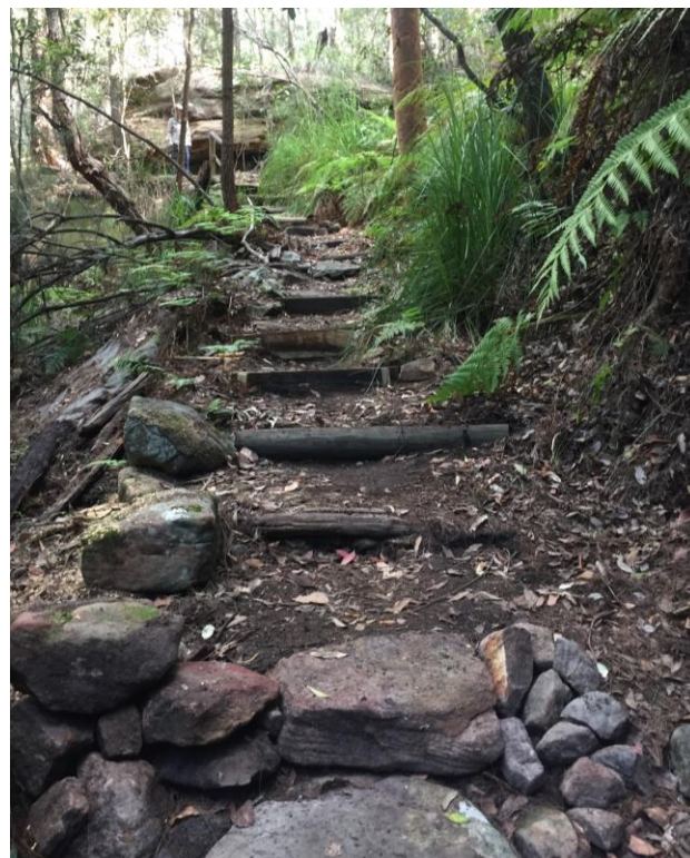
Repaired steps on the track leading up the escarpment near the beginning of the walking track.
